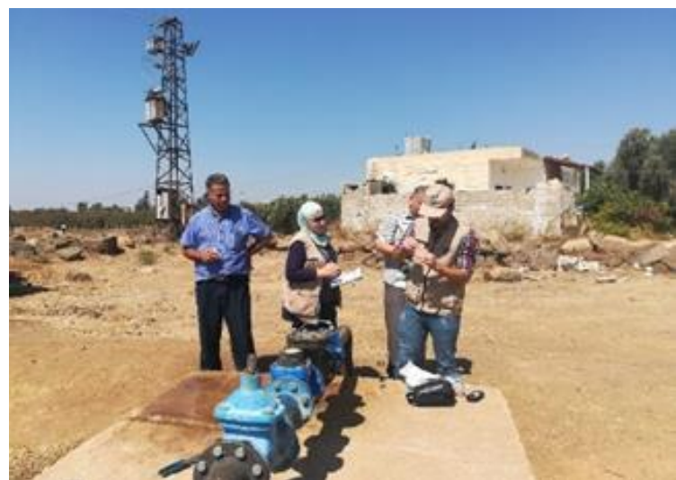
Water wells rehabilitated in Dara'a during a water quality surveillance visit by the local technical team
