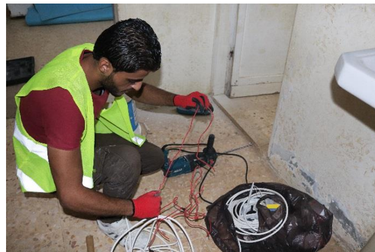
Training of local plumbers to install water-saving devices is a key aspect of the project.
