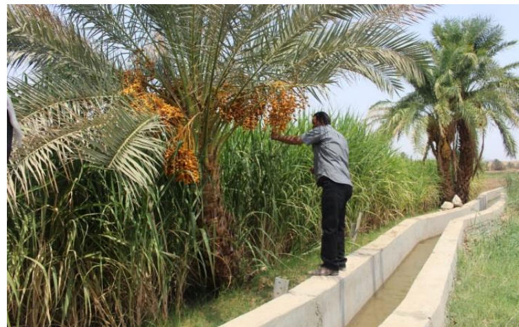
Rehabilitated irrigation channels helped reducing water losses and increased productivity of 1,275 farmers. © FDFA
